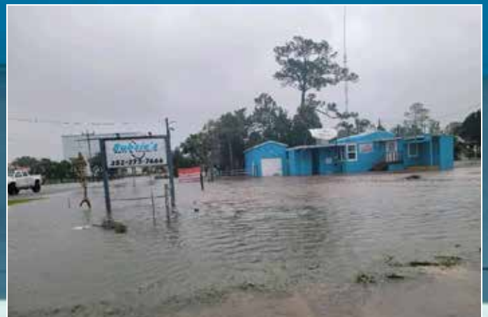
Flooding from Hurricane Debby.
